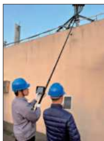
constructure inspection (WIFI real-time image transmission)
